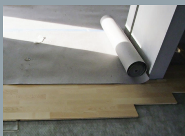
Peter Grønlund used DAFA Silence as an impact noise reducer throughout the house, which has floating floors.
