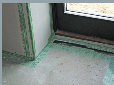
To meet the requirement of 100% sealed vapour barriers, DAFA Airstop System products were used for the seal.
